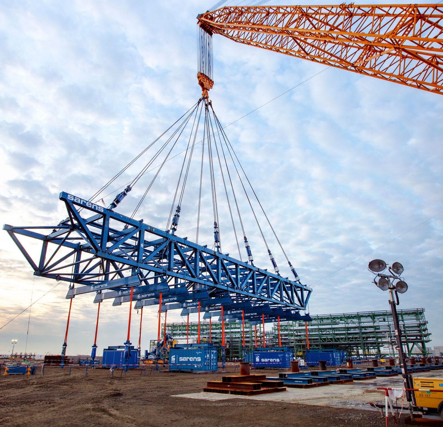
Photo: The Future Growth and Wellhead Pressure Management Project in Kazakhstan advanced in 2019 – all initial production wells were drilled, and pipe rack modules and gas turbine generators were installed.
