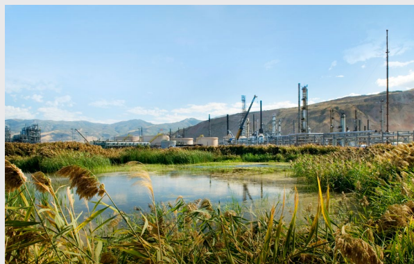
Photo: Chevron performed robotic inspections of in-service tanks at the Salt Lake City Refinery in Utah to collect asset integrity data without having to shut down the facility.
