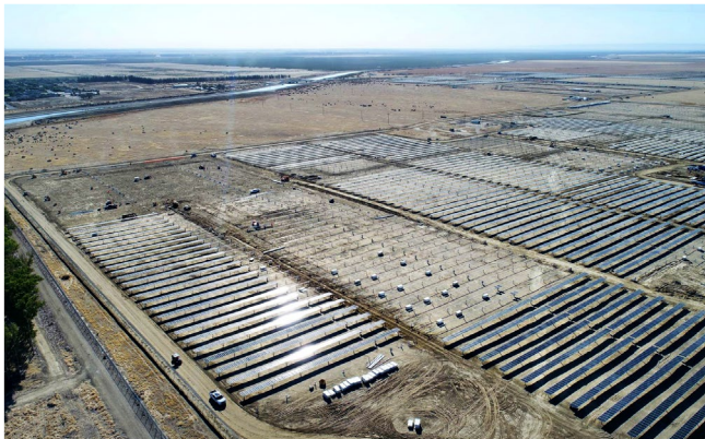
Photo: Construction is underway on a new 29-megawatt solar farm that is designed to supply 80 percent of the power needs at the Lost Hills Field in California.
