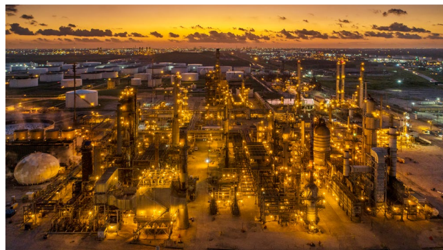
Photo: Chevron acquired the Pasadena Refinery in May 2019.
